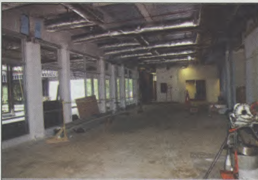
FORMER JAVA CITY STRIPPED BARE
